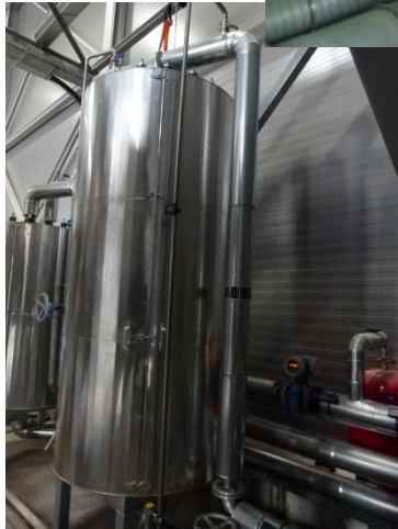
Spiral heat exchanger 260 kW
