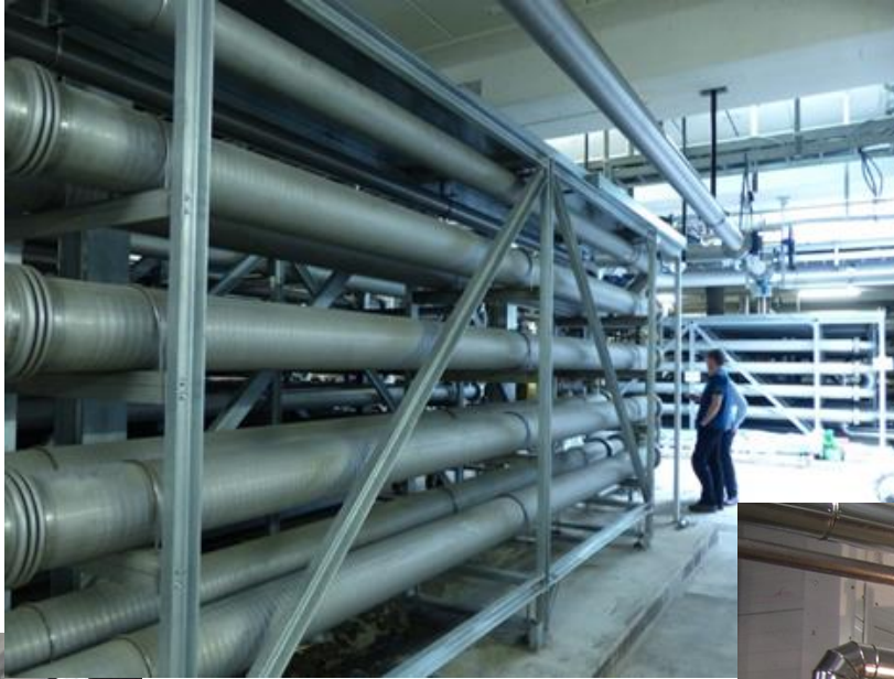
High performance pipe in pipe Heat exchanger 1900 kW
