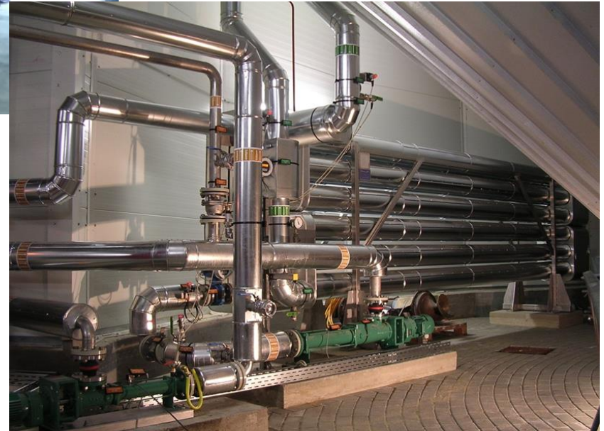
Conventional pipe in pipe heat exchanger 135 kW
